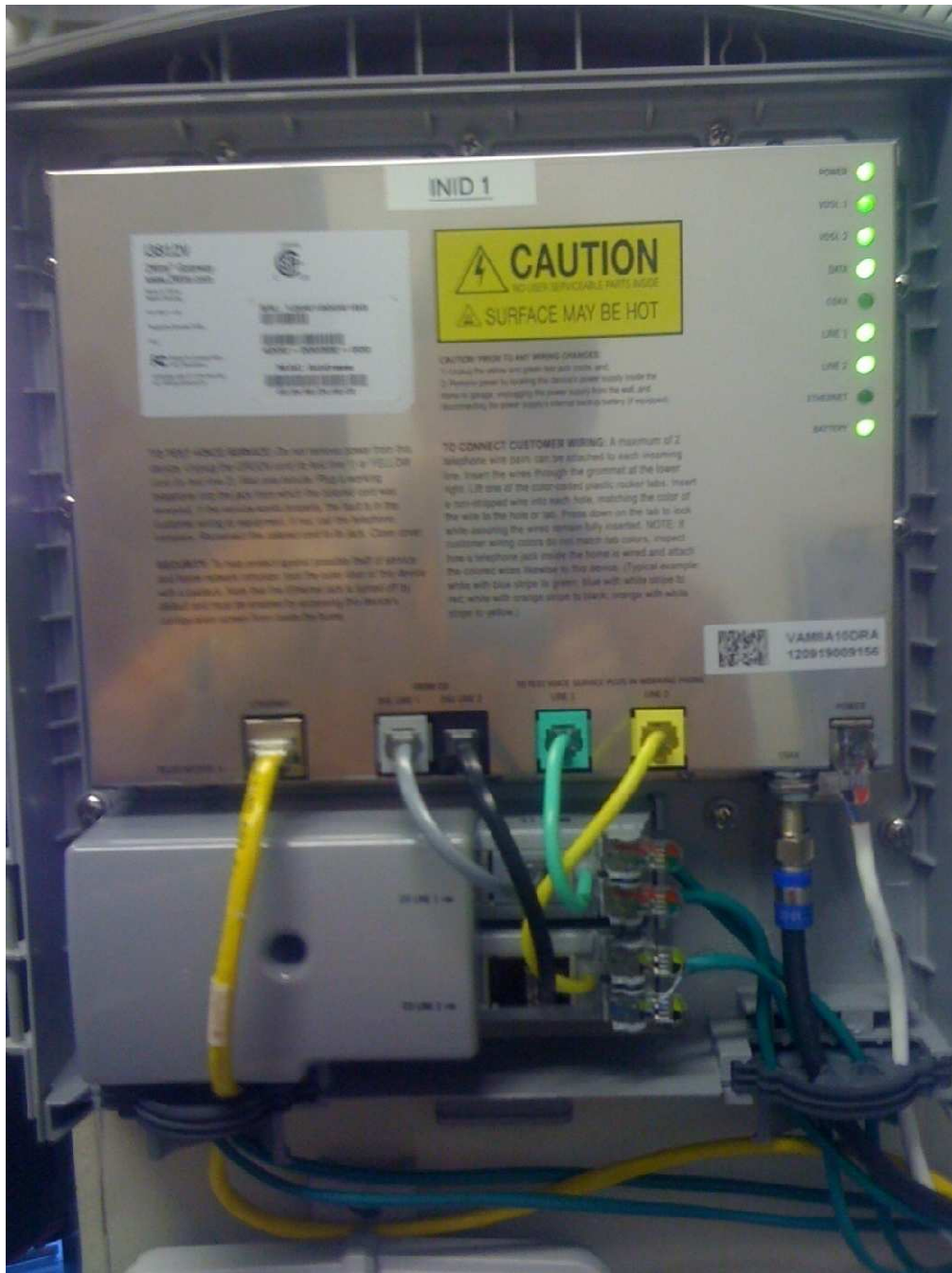
Figure 1. iNID Outside Unit with Cover Open
